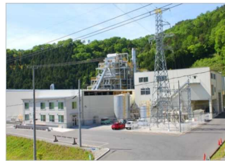
[Wood biomass power plant]
