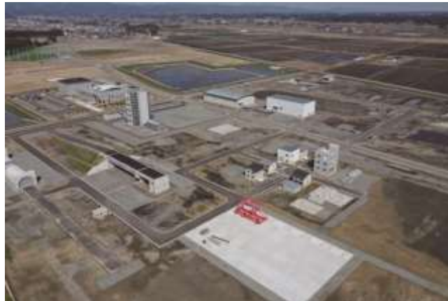
Figure Panoramic view of the Fukushima Robot Testing Field (industrial parks for reconstruction in Minamisoma City)
