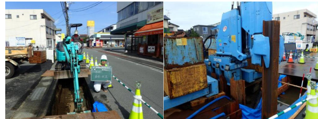
溝掘り部掘削
