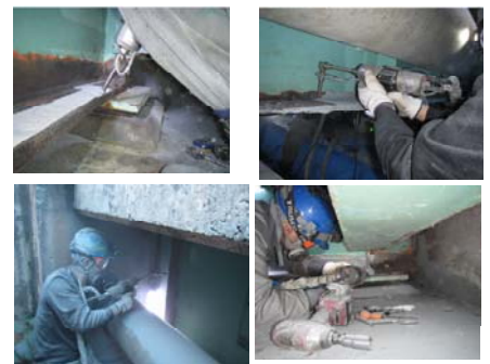
Photo 2 CS treatment under narrow space condition
