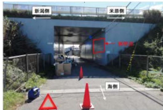
Fig.5. Experiment scenery in a box culvert at Hokuriku highway.
