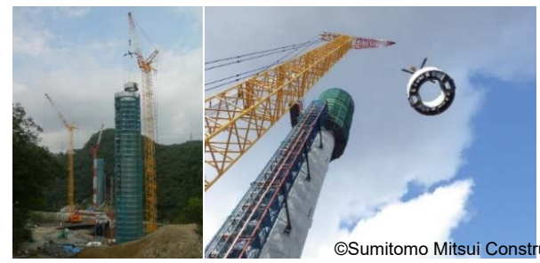
Hung and placed with a crane
