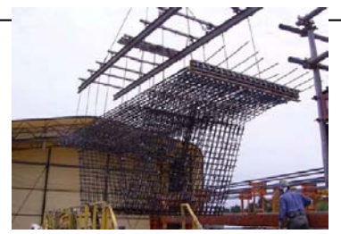
Prefabricated rebars
