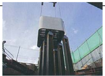
Bridge bottom Embedded formwork of piers
