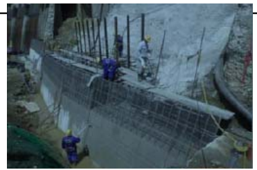
Retaining work Embedded formwork of external walls
