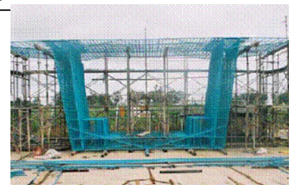
Prefabricated rebars
