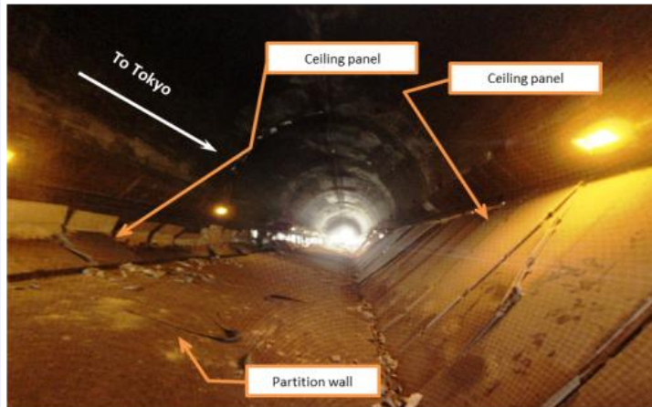
Sasago Tunnel (east bound) to Tokyo
