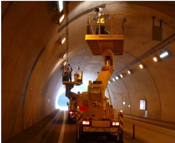
Inspection of tunnel equipment
