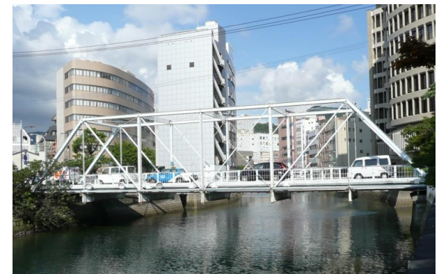
Dejima Bridge (Nagasaki Pref.) Built in 1910 (about 102 years old)
