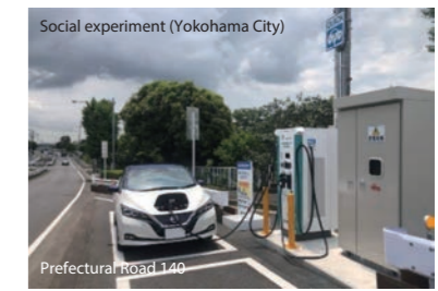
Installation of EV charging facilities on public roads
