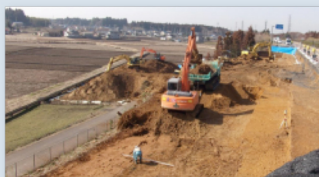
Work efficiency enhanced by borrowing adjacent land
