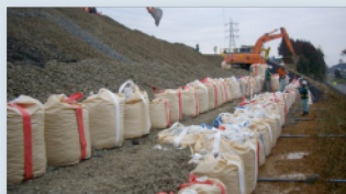
Shorter work period owing to carefully selected materials (crushed stone)
