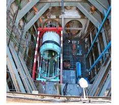
Method to install sewerage pipes without excavating the road (left in the center of photo)
