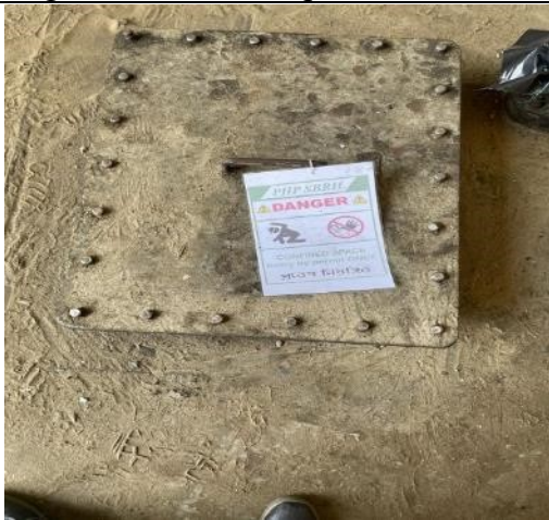
Installation of laminated warning labels
