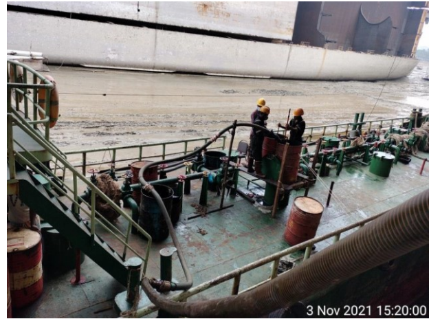
The work of extracting residual oil
