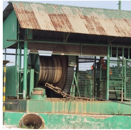
Winch installed inside the yard
