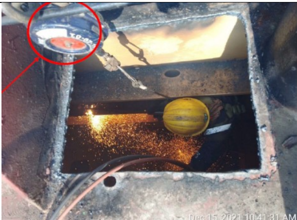
Installation of fall prevention gears for work in high places
