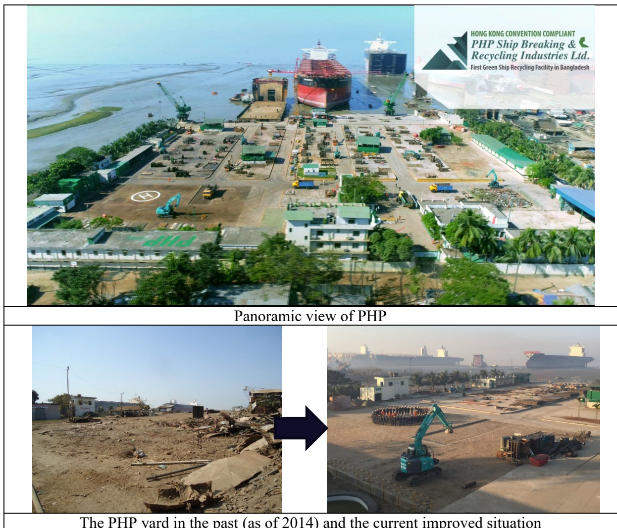
Figure 4-1 Panoramic view of the PHP yard
