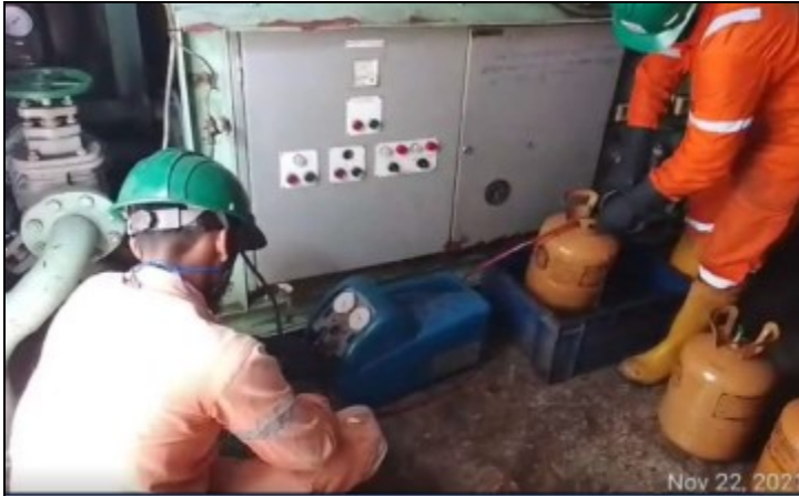
ODS removal work
