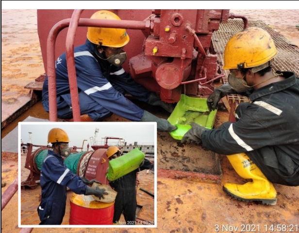
Waste work oil removal work
