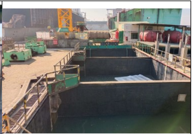
Waste water treatment facility
