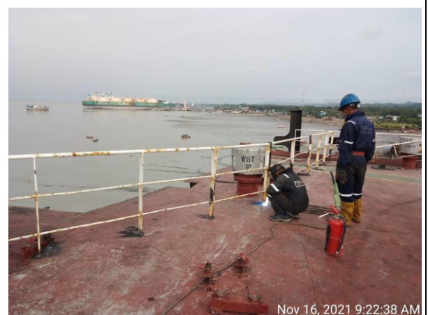
Installation of fall prevention fences (work in high places)
