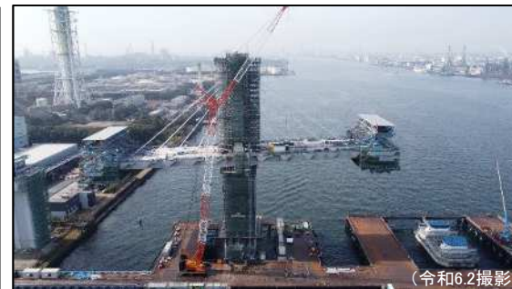
②主橋梁部MP1～MP3
