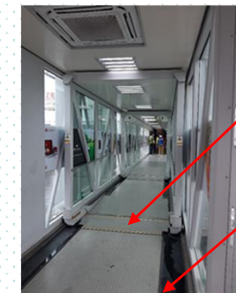
Steps Inside Standard PBB Tunnel
