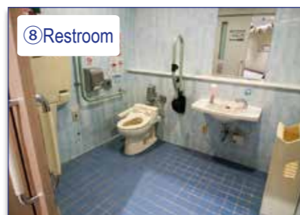
⑧ Restroom Accessible restroom on the same floor Handrail: Movable (L) / Fixed (R)
