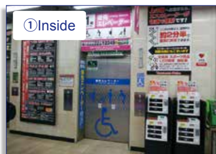
① Inside Accessible elevator
