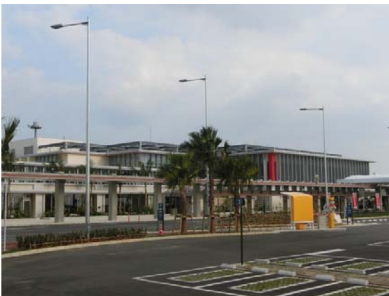
Terminal building at the newly opened New Ishigaki Airport (photograph supplied by Ishigaki Air Terminal Co., Ltd.)
