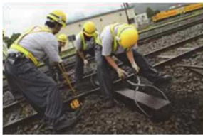
Repair of railway facilities
