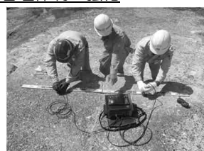
護岸の点検・補修
