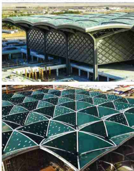
〈MEDINAH STATION ROOF:2012〉
