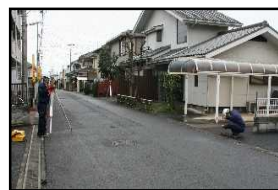
[現況測量の様子]
