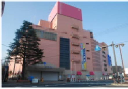
Exterior appearance of new Ishinomaki city government office
