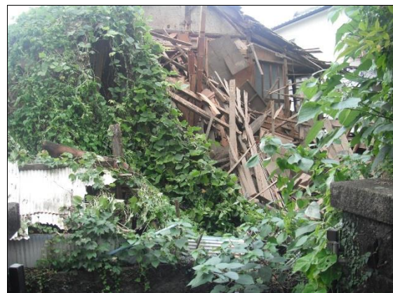
A dilapidated empty house (above) and a produced open space after its removal (below)
