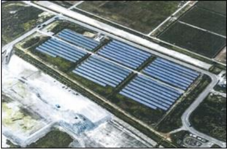
Source: Material of Higashi-Matsuyama city
