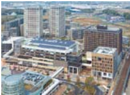
Kashiwa-no-ha Smart City, realizing energy efficiency through cooperation with communities
