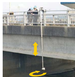
P C桁の点検
