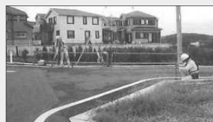
[現況測量の様子]
