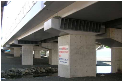
< 橋梁の耐震補強 >
