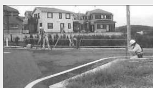
[現況測量の様子]
