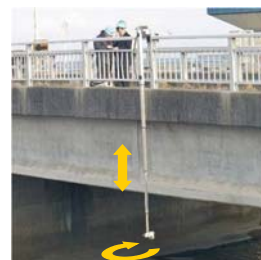
P C 桁の点検
