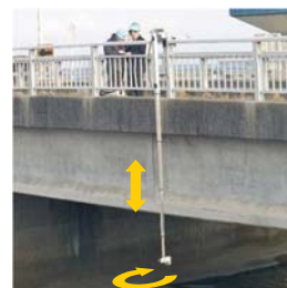
P C 桁の点検
