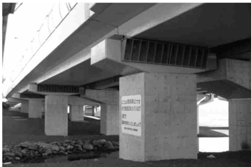
< 橋梁の耐震補強 >
