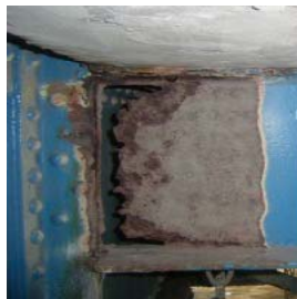
H21損傷状況 (主桁腐食)
