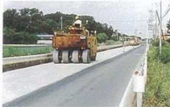
Applying seal coat
