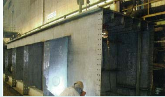
Assembled into Girder
