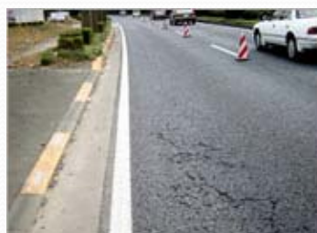
Removal of damaged pavement
