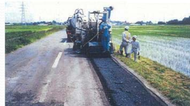
Cold in-place surface recycling
