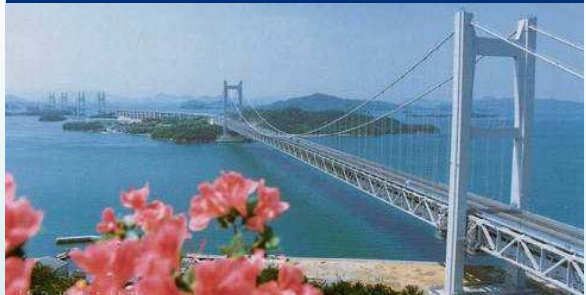
Shimotsui-Seto Bridge (1988) Okayama Pref.
