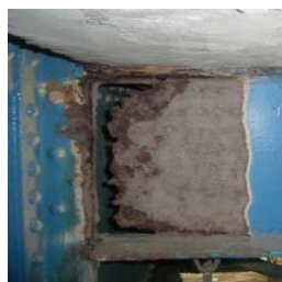
H21損傷状況 (主桁腐食)
