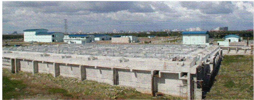
Sewage treatment in HCM (141,000 m 3 /day, completed in 2009)
