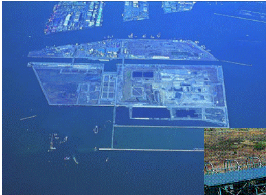
Leachate Treatment in Central Breakwater Landfill Site (20,500 m 3 /d)
