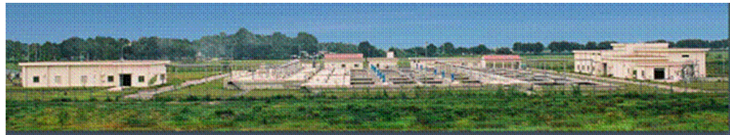
Sewage treatment in in Thang Long North (42,000 m 3 /day, completed in 2008)
