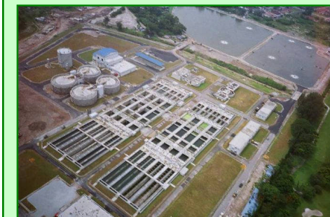
Kuala Lumpur City sewage plant (5 places, Treated quantity: 250,000m 3 /d)
