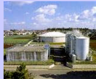
Water distribution Plant*2
