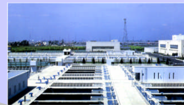
Municipal water treatment plant
