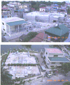
Advanced sewage treatment in Hanoi CP-12 (2,300 m 3 /d & 3,700 m 3 /d, 2005)
