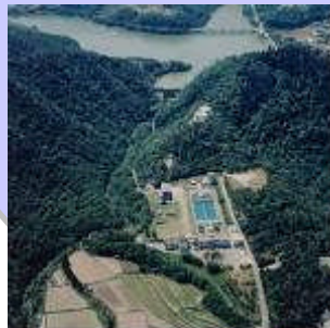
Intake water facility*1
