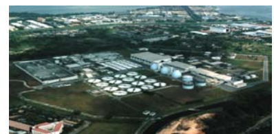
WWTP in Singapore (75,000 m 3 /d)
