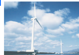
Offshore wind power generation facility in Setana, Hokkaido
