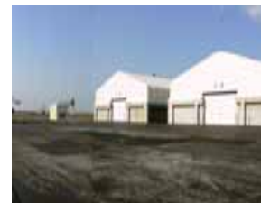
汚染土壌等保管施設 (酒田港)
