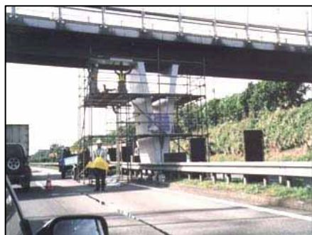
橋梁の耐震補強
