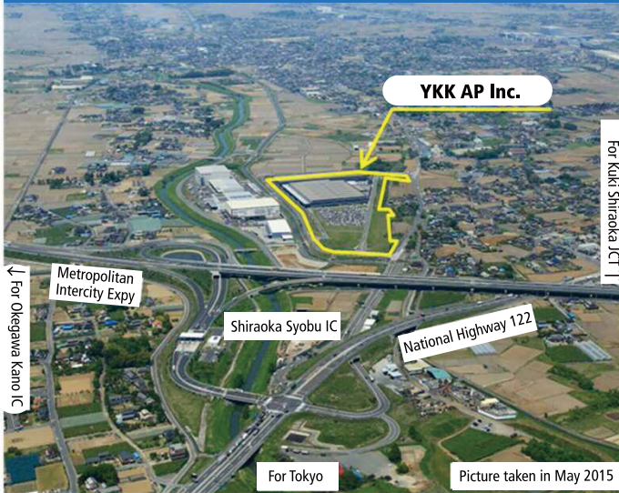
A window manufacturing factory near Shiraoka Shobu IC
