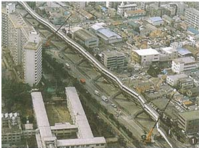
Damage caused by the Great Hanshin Earthquake
