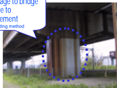
Photo: Bridge piers (Tokamachi district, Nagaoka City)
