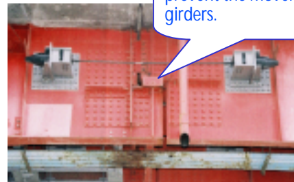
Photo: Aseismic connector (Wanatsu district, Nagaoka City)
