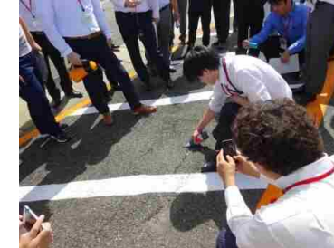
ひび割れ補修剤注入を実演
