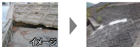
ひび割れ補修
