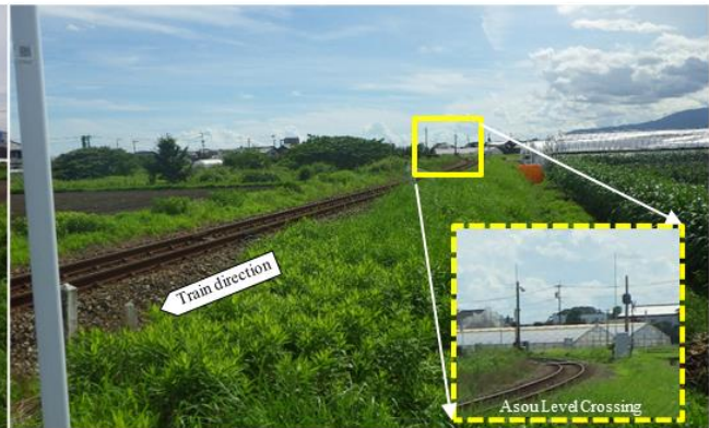
Sighting status of direction to Nishi-Tachiarai station viewed from the entered side of the light motor vehicle
