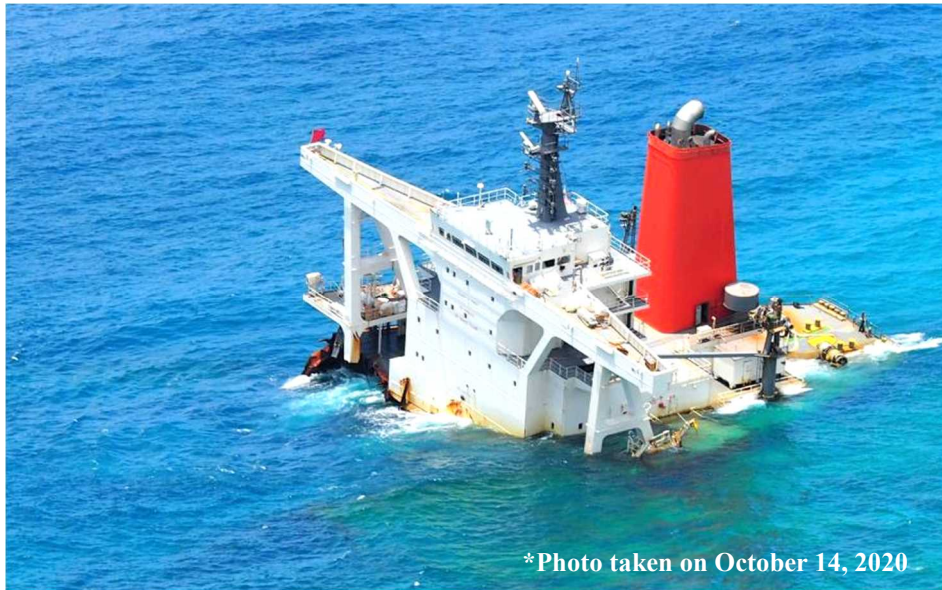
Photo 10 The Broken Hull (Stern Portion)
