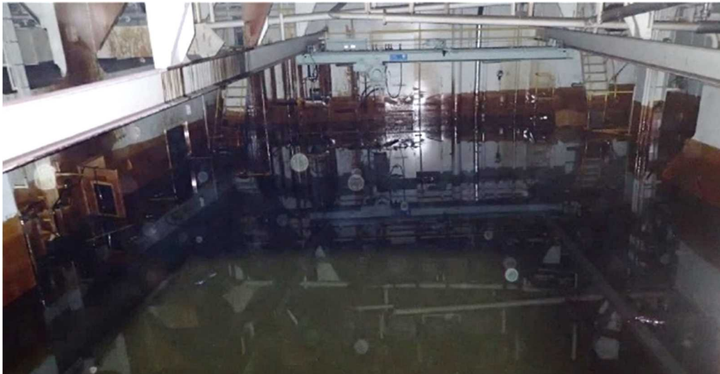
Photo 3 The Flooded Engine Room
