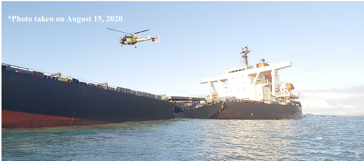
Photo 6 The Broken Hull
