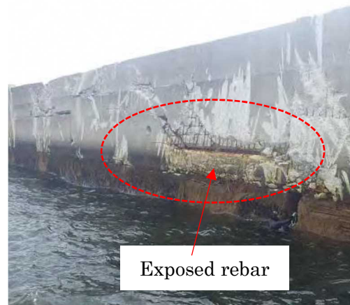
Gouges and abrasions in the concrete
