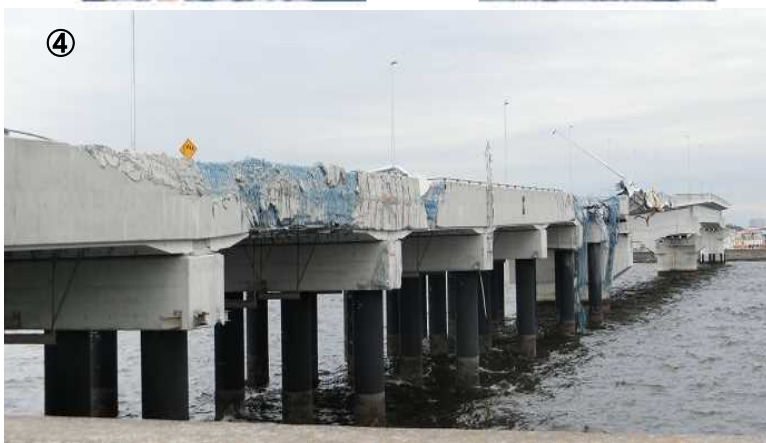
Prestressed concrete pier
