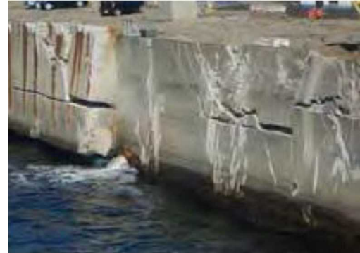
Gouges and abrasions in the concrete
