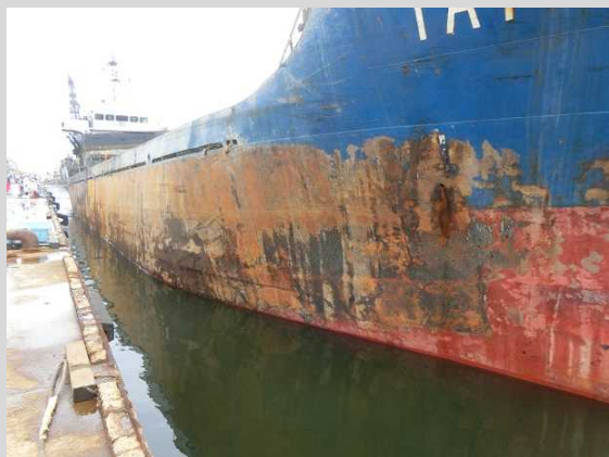
Starboard plating shell
