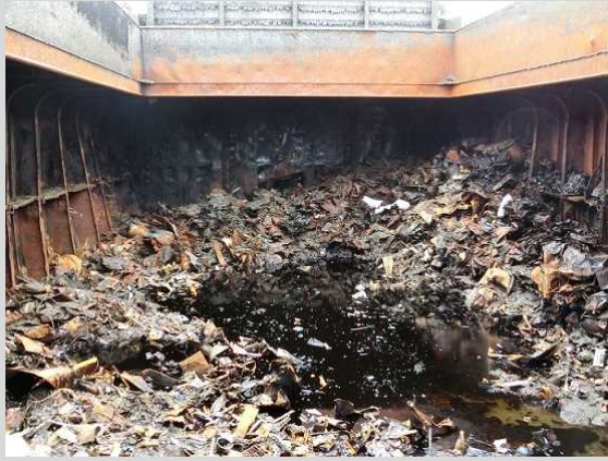
Aft side of the Cargo Hold
