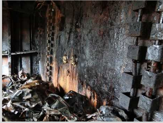
Aft-side bulkhead of the Cargo Hold
