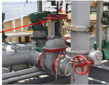
(Photo 2.5-5 Bypass valve operation handle)
