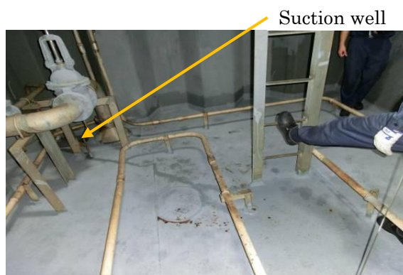
Photo 2: Bottom of No.2 cargo tank (port side)
