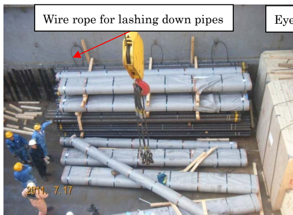
Photo 2.1-4 Wire Rope for Lashing down Pipes
