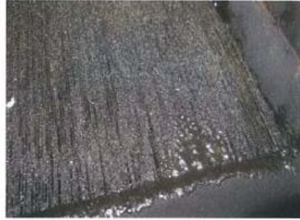
Soiling of the air side of the air condenser of the stand-by diesel generator
