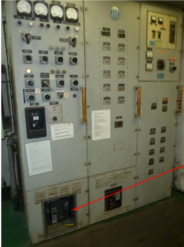
Photo 5: Emergency Switchboard
