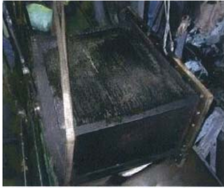
Soiling of the air side of the air condenser of the stand-by diesel generator
