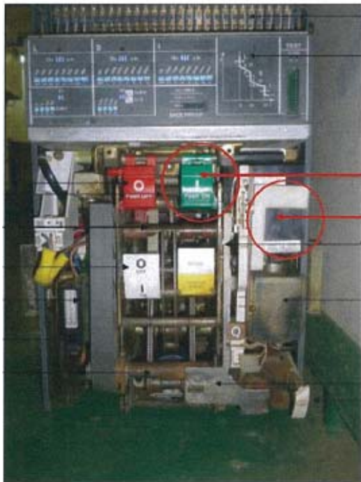
ACB for the emergency diesel generator (The ACB is removed from the generator)
